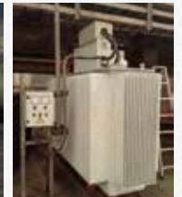
Replaced APL No. 4 electrolytic rectifier transformer
