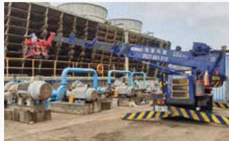
Protection for elevated work activities
