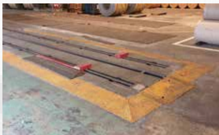
Ground leveling work
