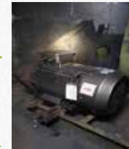
Replaced high efficiency motors for the jet cooling fans used at the APL cooling section
