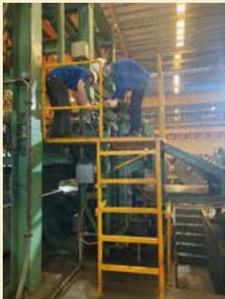
Setup of elevated maintenance platform
