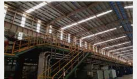
Railings for work stations in the pickling section of APL
