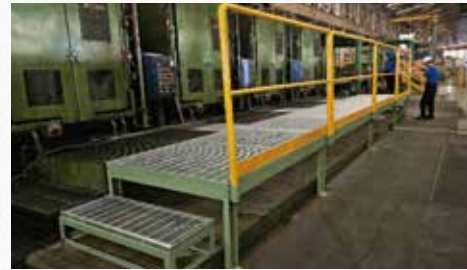
Installation of railings at the job site
