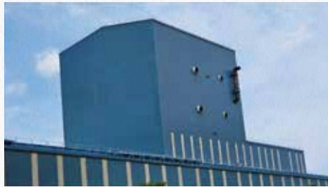
Setup of guardrails around the roof of the factory
