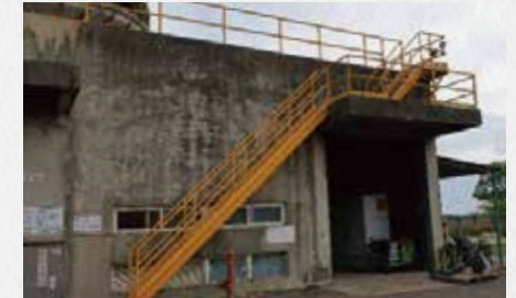
Outdoor ladders replaced with stairs
