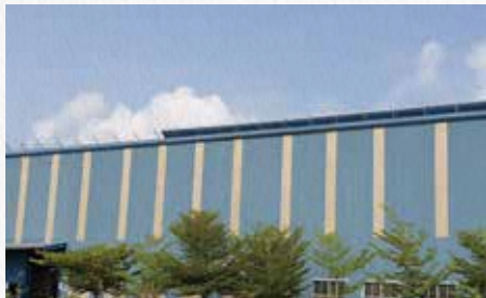
Installation of new protective rails around the rooftop
